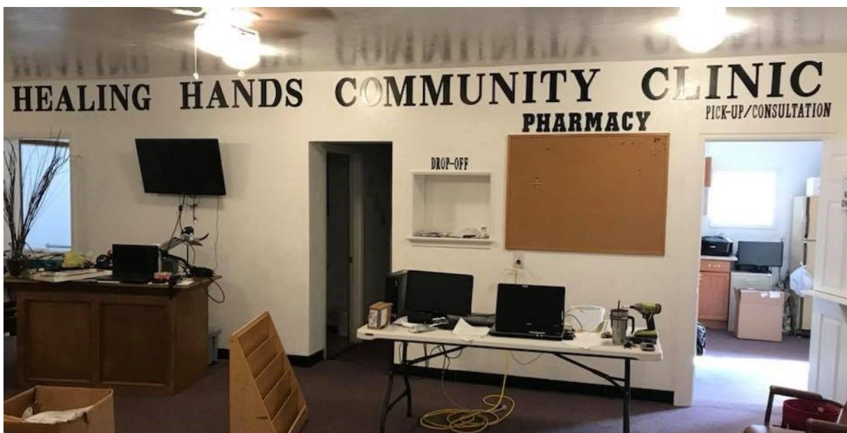
Healing Hands Community Clinic – Under Construction August 2018
